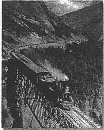
▲ A railroad bridge in the American West. Oil over a photograph, circa 1870.
